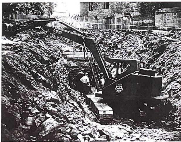
Jack Shannahan Overseeing the Digging of the Mine Entrance, circa 1972
